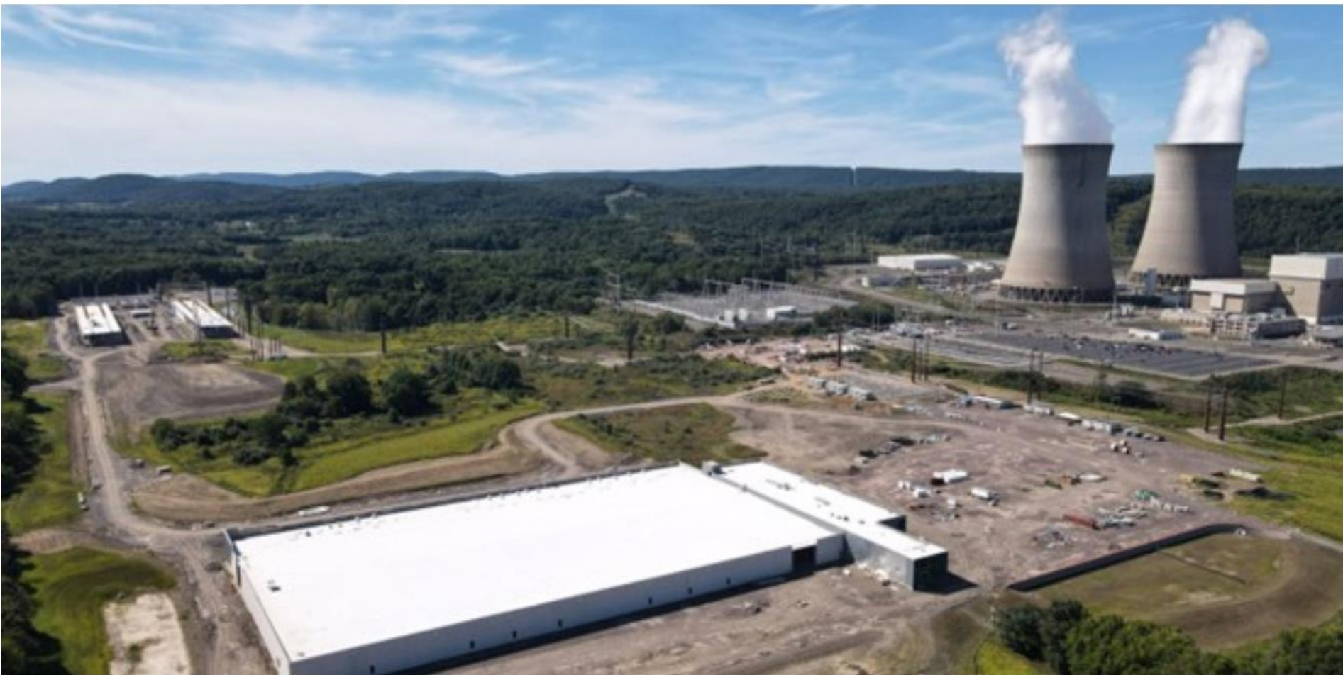
Susquehanna nuclear plant in Salem Township, Penn., along with the data center in foreground. (Photo: Talen Energy)
